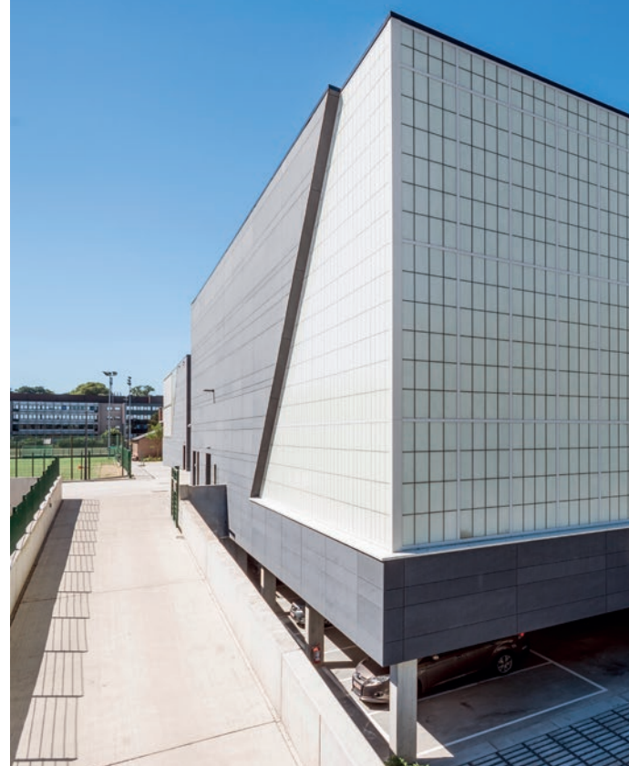
▲ The translucent wall panels bring in a lot of daylight and make for a unique facade.
